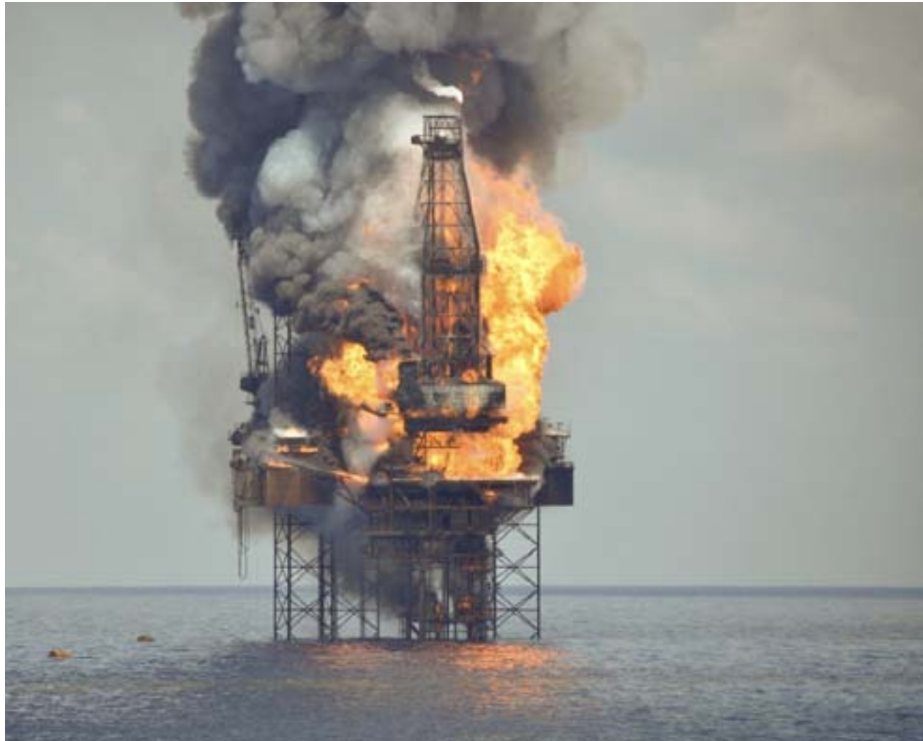
▲ Montara rig and platform on fire
